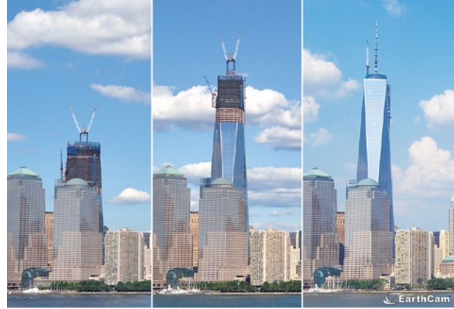
EarthCam technology helps share construction project progression such as One World Trade Centre in New York City. - Photo: EARTHCAM
