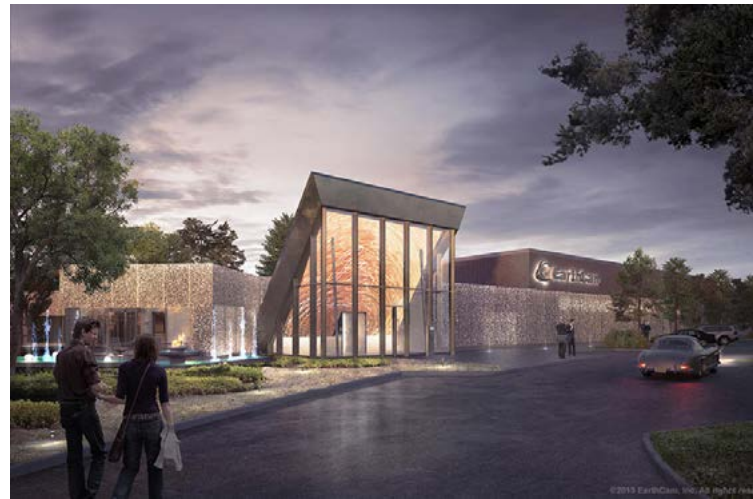
This is a rendering of EarthCam’s new offices to be located in Saddle River. | Courtesy Earthcam
