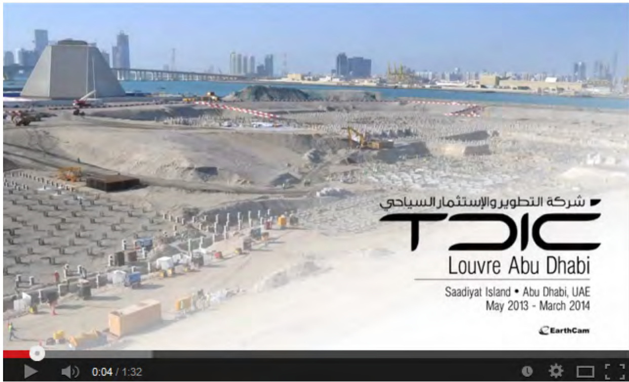
The progress in construction of the Louvre Abu Dhabi museum on Saadiyat island in the last eleven months, depicted in a time-lapse.
