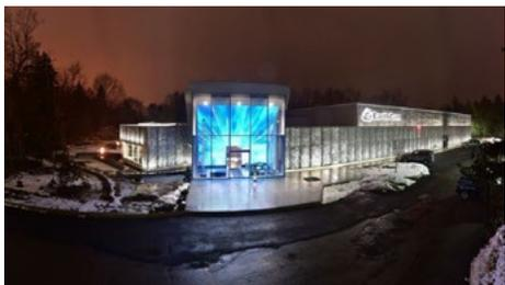
Translucent aluminum foam panels framing 25-foot-tall LED video wall at EarthCam's new headquarters (Joe Kitchen)
